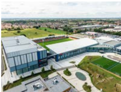
LNER York Community Stadium
