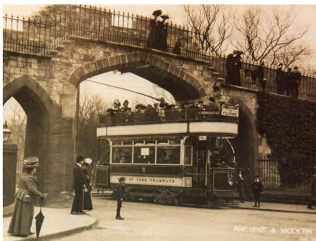
**2.26** The Rougier Street archway, as raised in 1906 to permit the passage of double-decker trams. The inserted masonry is clearly visible in the arch (Private Collection).
