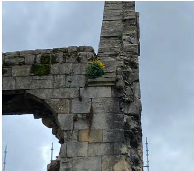
Structural movement to gable junction with wall
