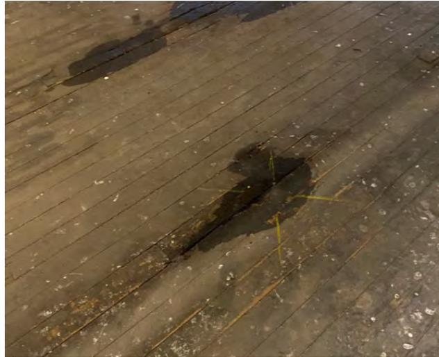
Multiple areas of water ingress from roof onto timber structure below
