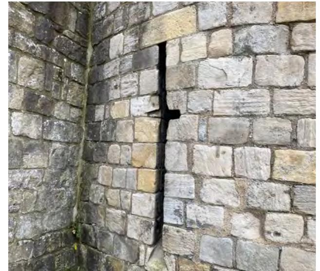
Structural movement to joint with east wall
