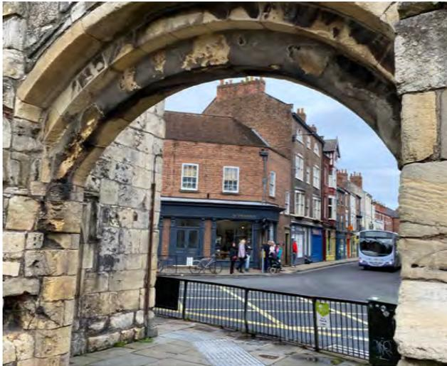
Erosion of stone from water getting trapped behind sulphuric crust
