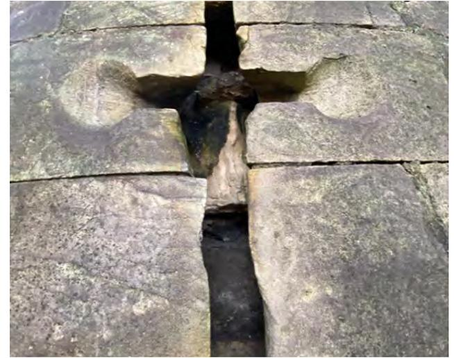
Masonry infill to interior of tower
