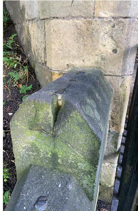
Rust jacking to removed railings
