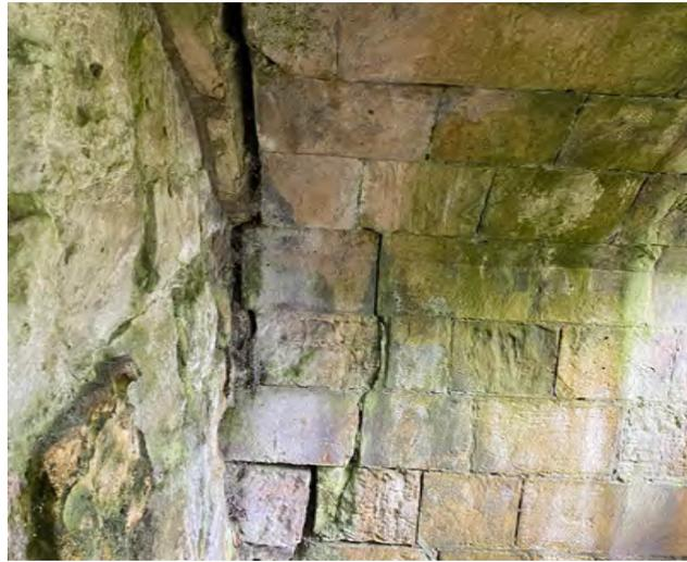
Joint failure between Victorian and Medieval structure
