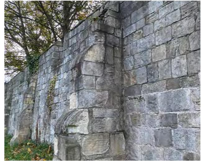
Missing masonry from buttress east of Robin Hood Tower
