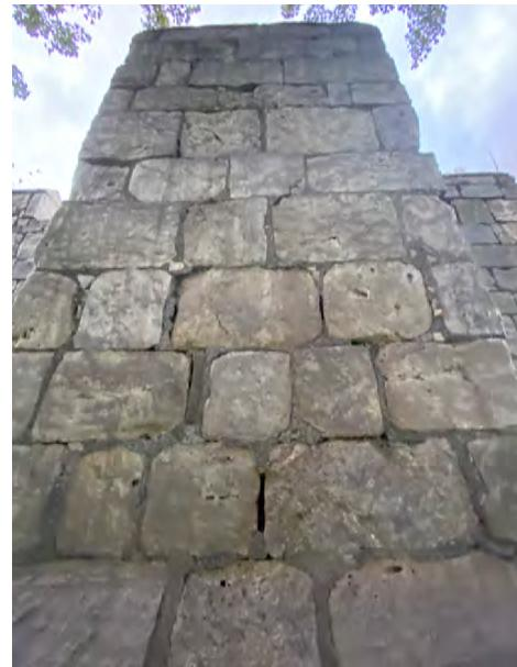
Structural cracks and open joints to southern elevation
