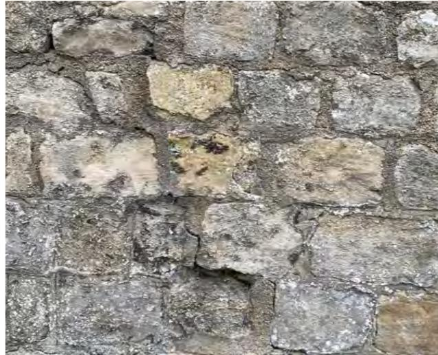
Diagonal cracking to wall on the west side of tower
