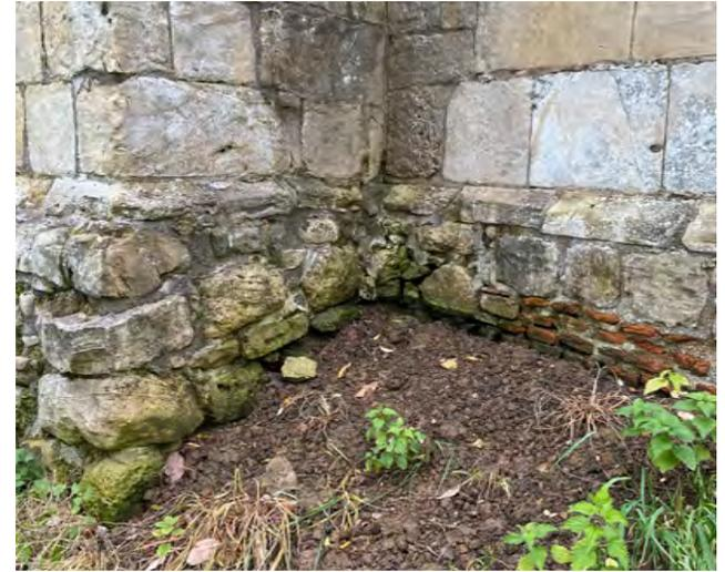
Rubble foundations are failing
