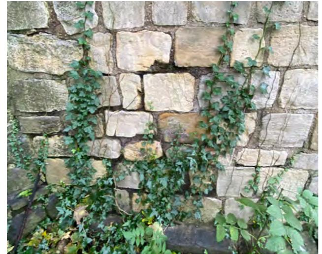
Saturated masonry at low level with failing mortar
