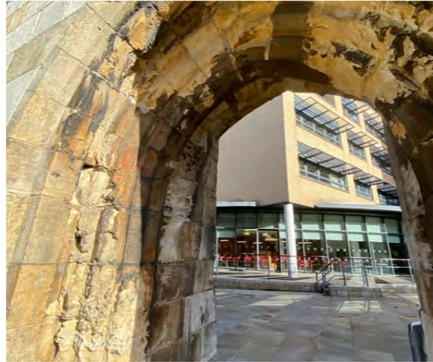
Heavily weathered stones to Victorian pedestrian arch between railway arches
