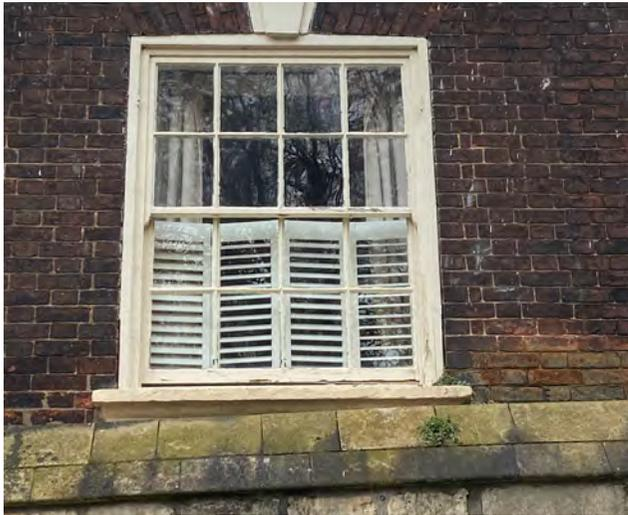
Erosion of water within brick above low level stone
