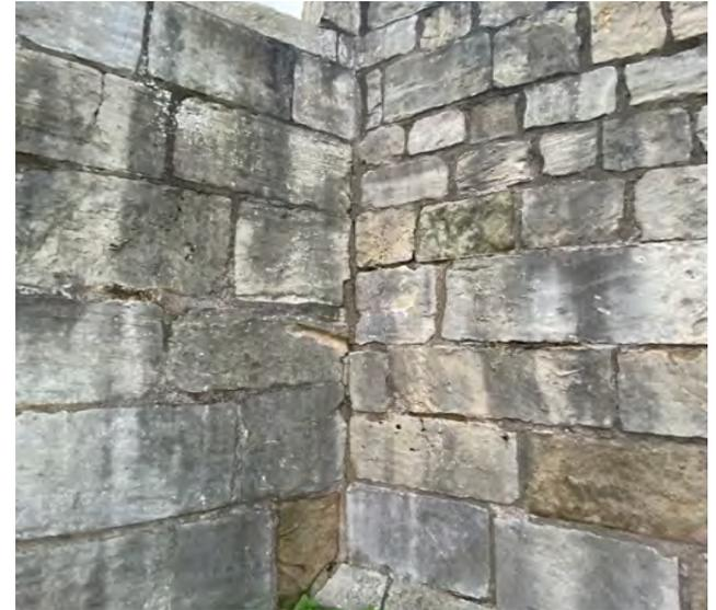
Movement crack to eastern junction with wall
