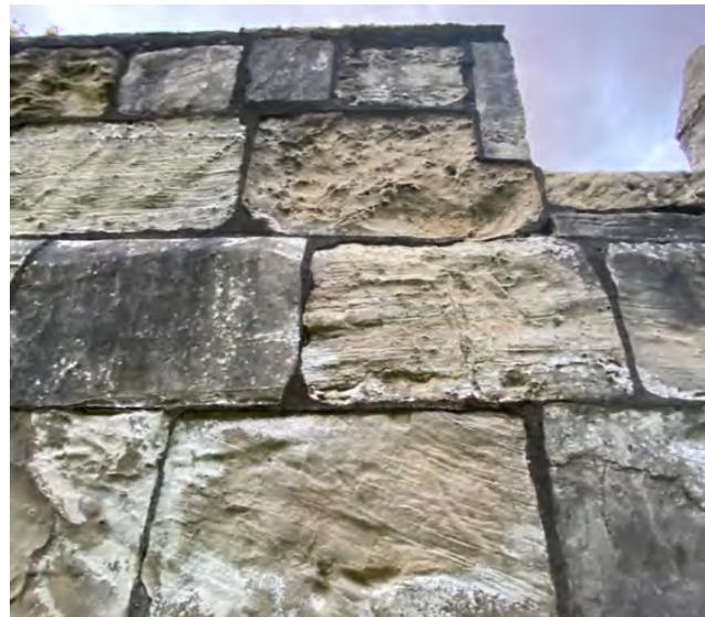
Poor hard cement mortar at Fishergate Postern Tower end
