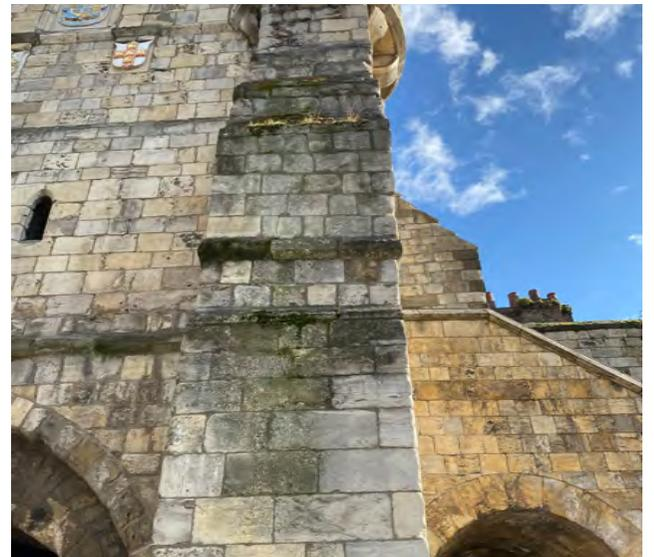
Structural movement cracks running up tower
