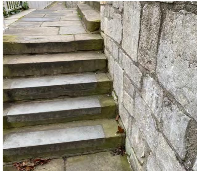
Walkway steps, enlarging joints against parapet wall
