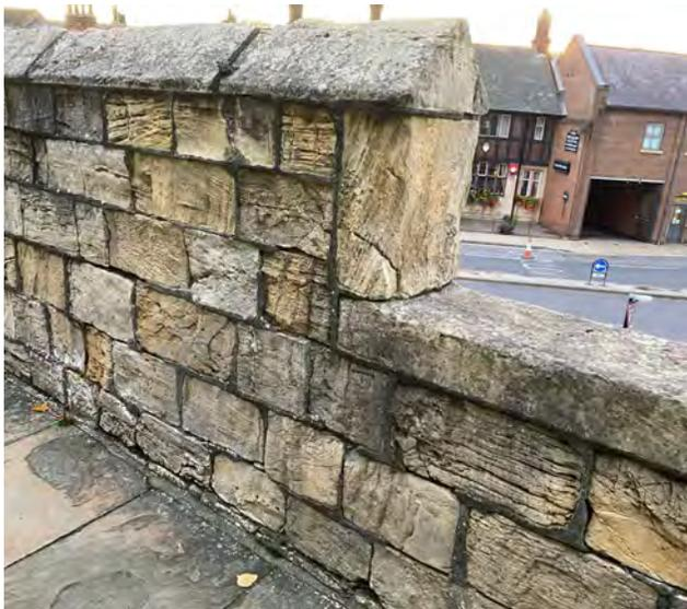
Fishergate Postern Tower end poor parapet wall condition
