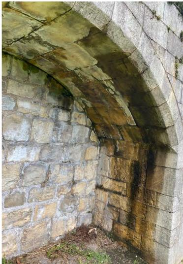
**3.15** Salt Movement and Saturated Masonry
