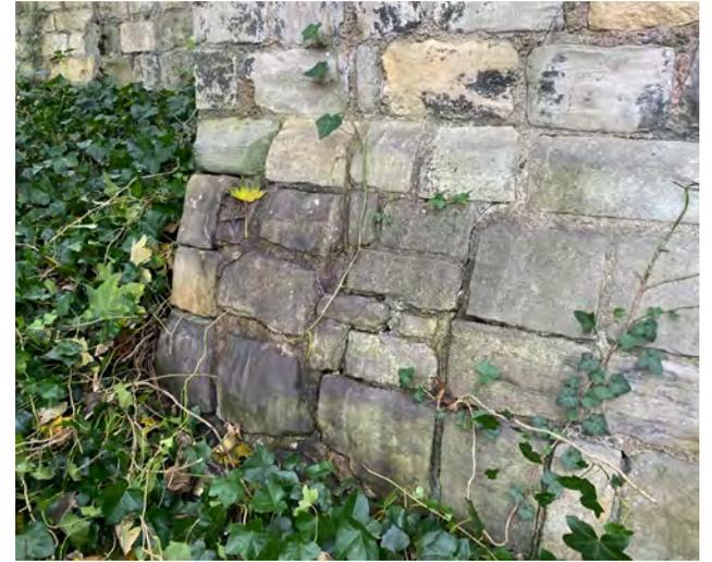
Spreading at corner foundations
