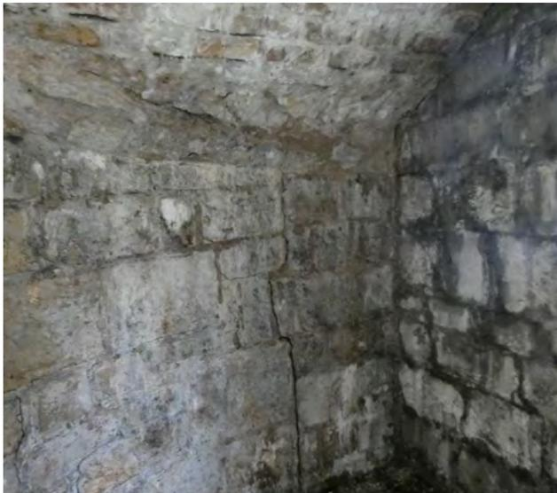
Structural movement to internal walls
