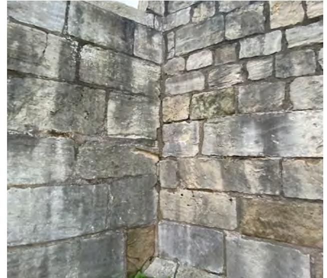
Movement crack to eastern junction with wall
