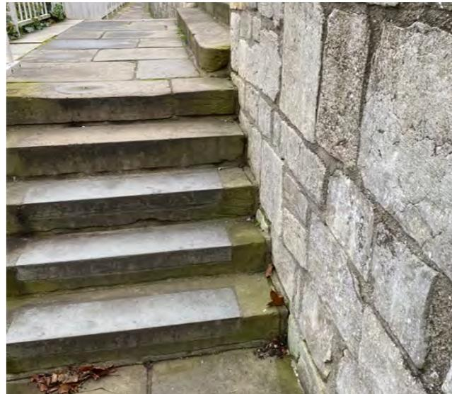
Walkway steps, enlarging joints against parapet wall
