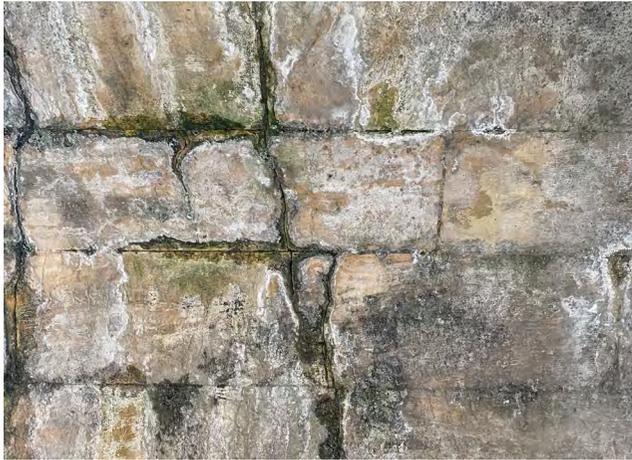
Cracks along stone arches
