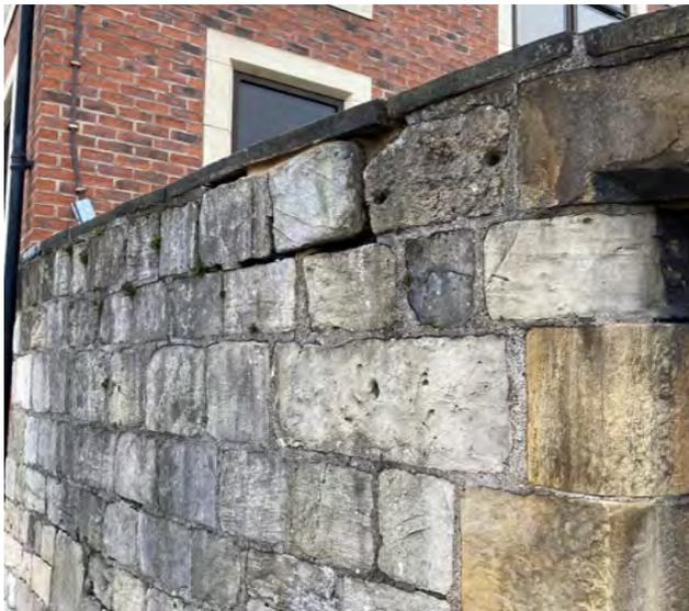
Open joints to low perimeter wall
