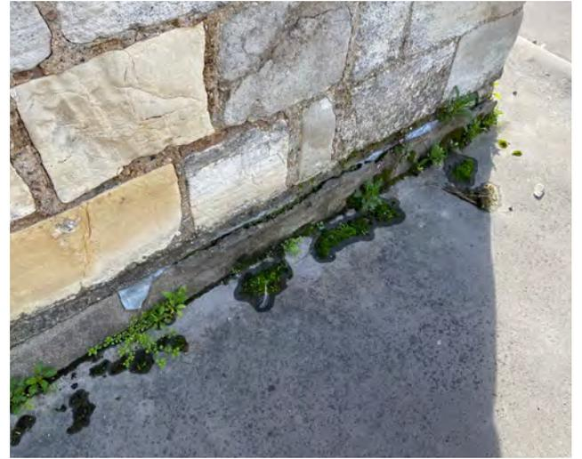
Missing lead and failing junction between asphalt and walls
