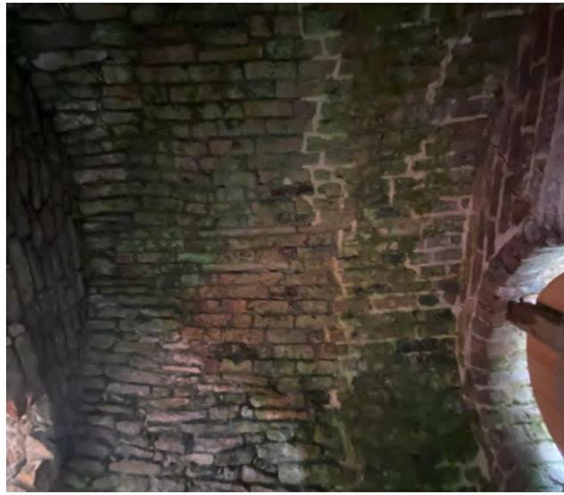
Structural movement cracks to brick barrel vault
