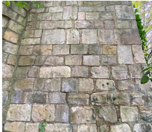
Vertical cracks to north elevation
