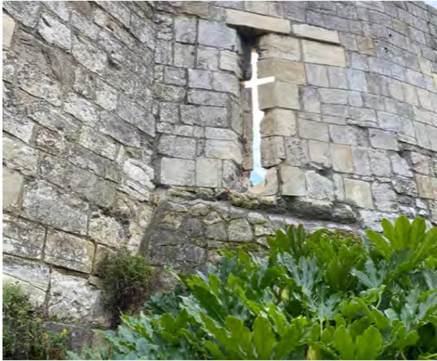
Failing cementitious mortar to north junction
