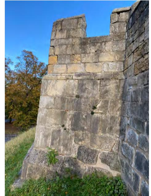
Structural cracks to south west elevation
