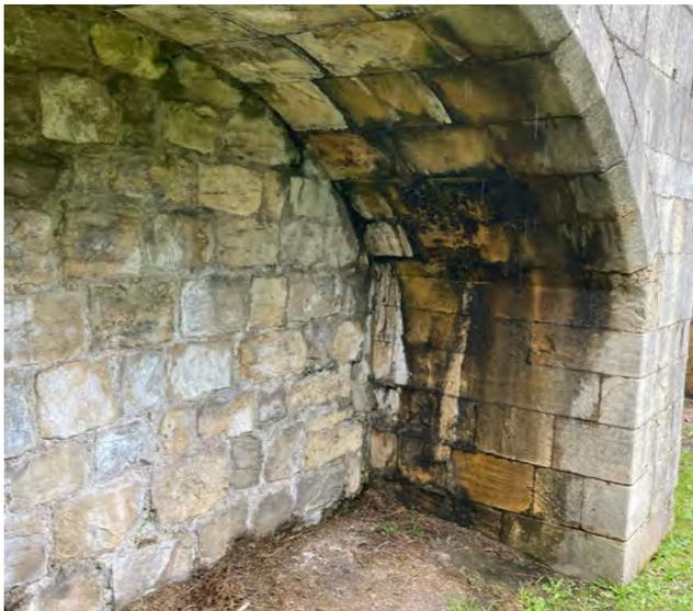
Saturation to interior of internal arches
