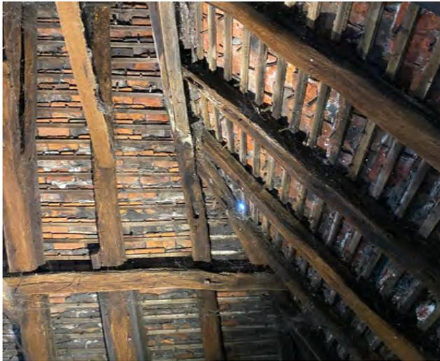
Holes in clay tile roof and rotting timber roof structure
