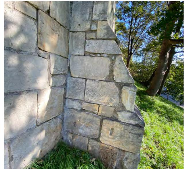
Structural movement to buttress 25m chainage
