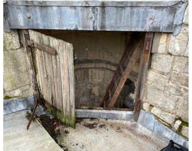
No covering to access hatch to roof which is allowing water in
