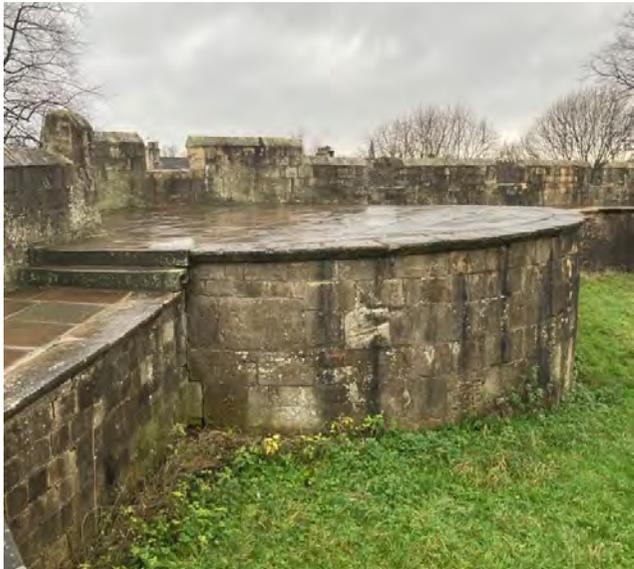
Cracking to east junction with wall
