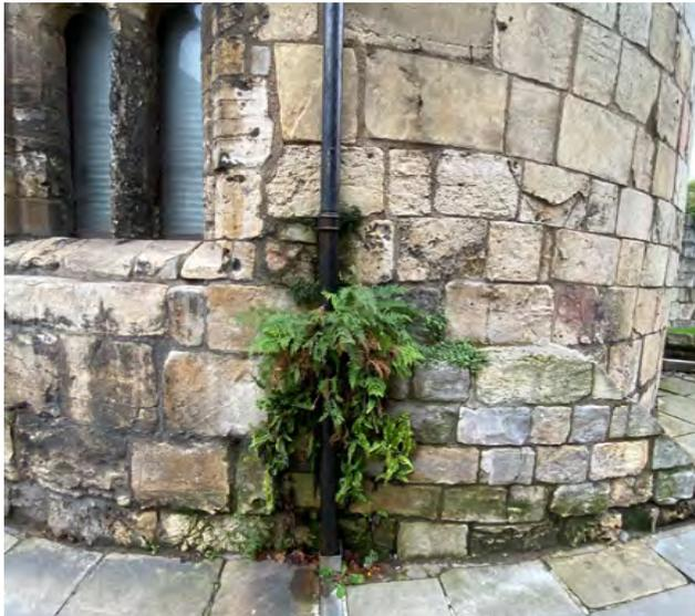
Leaking rain water pipe
