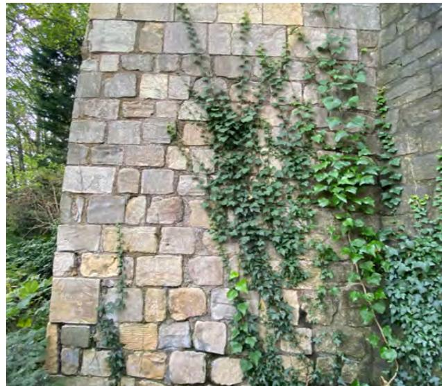
Vertical cracks to southern elevation
