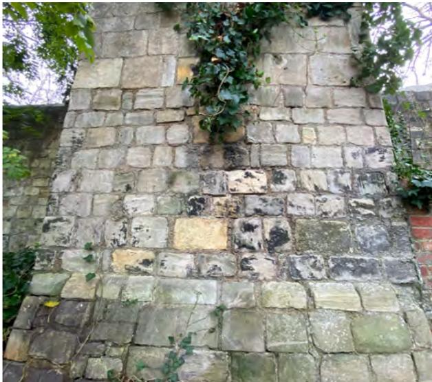
Vegetation growth and open joints to west elevation
