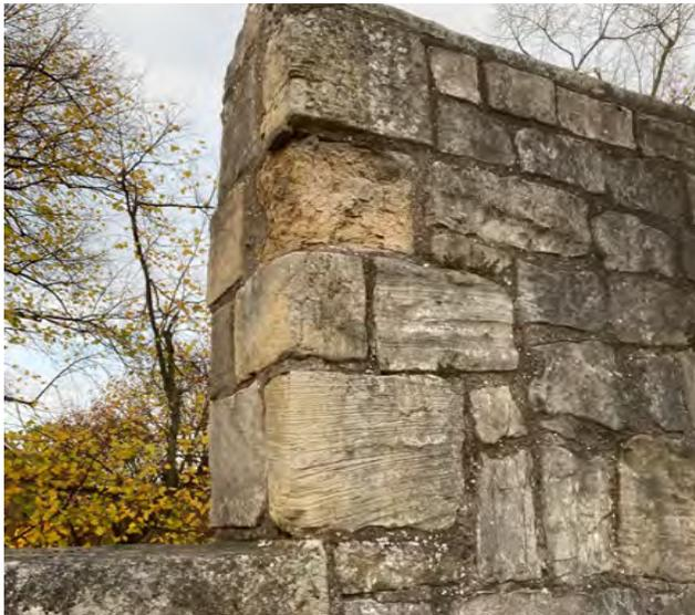
Eroding stone to merlon
