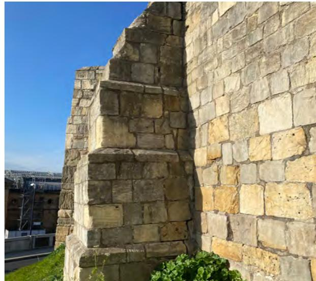
Structural movement to buttress next to Tofts Tower
