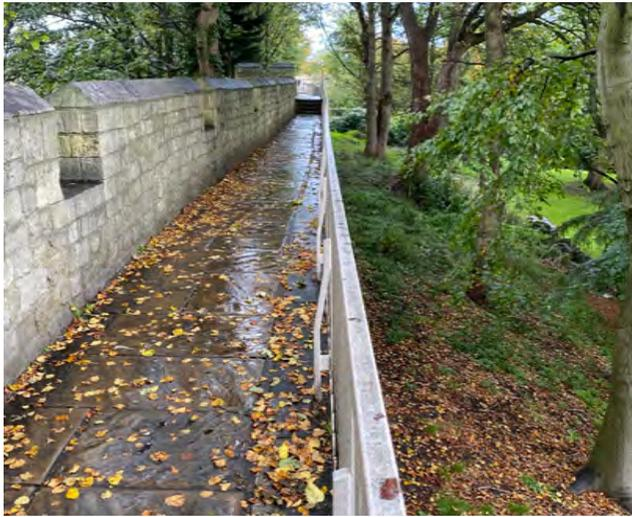
Bending railings with no movement joints
