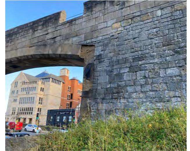
Spalling stone from rust jacking from concentrated water
