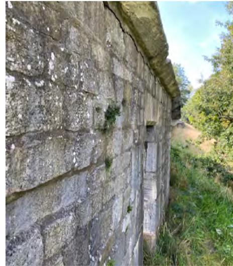
Mortar joint below edges stones moving outwards
