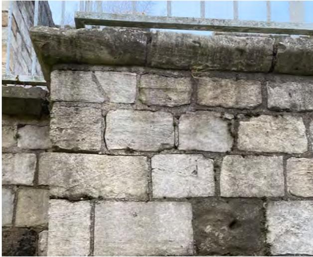
Cracking and open joints to western walkway structure
