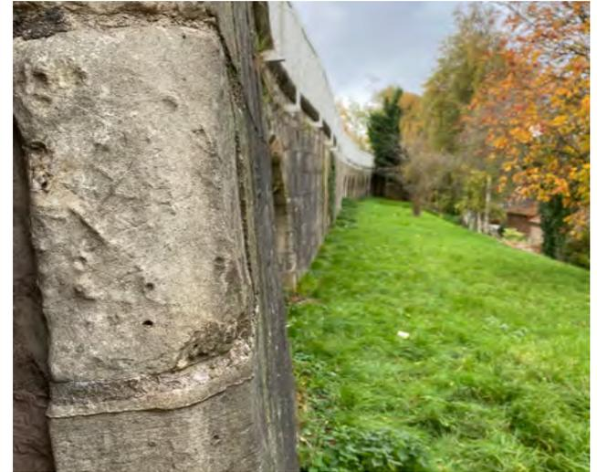
Internal wall below walkway is at an extreme angle
