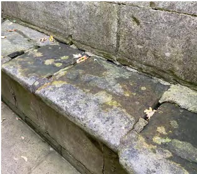
Failed concrete mortar and open joints to walkway
