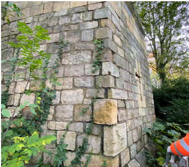
Separation of masonry around the quoins of tower
