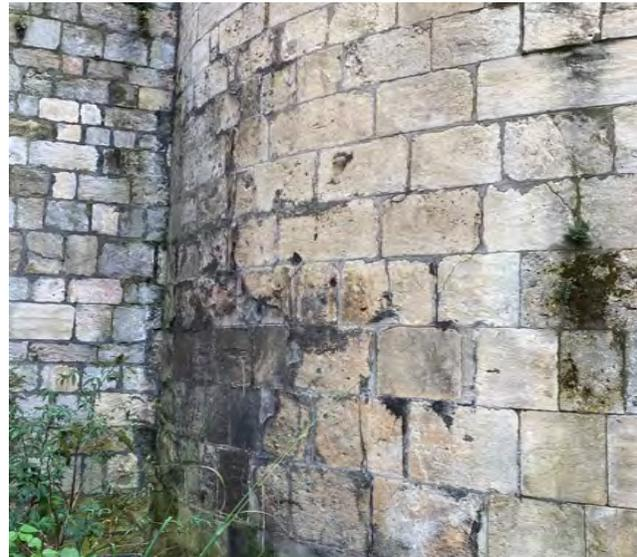
Structural cracks, fractured stones and failing cement mortar to eastern junction with wall
