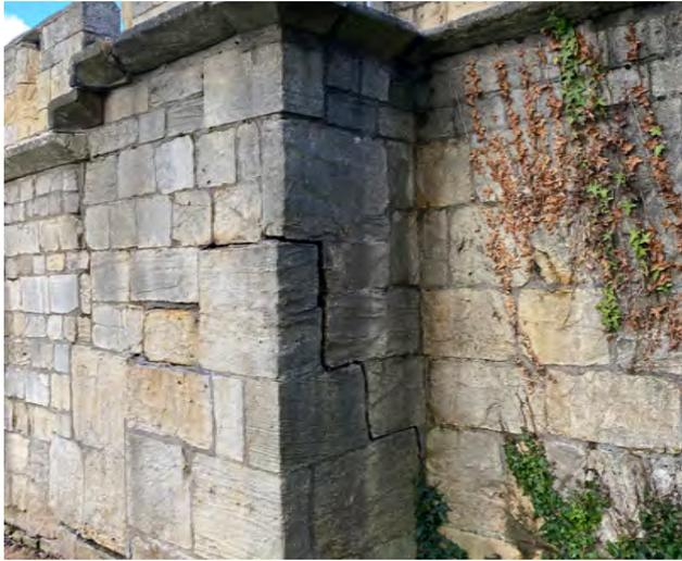
Cracking below steps and railings
