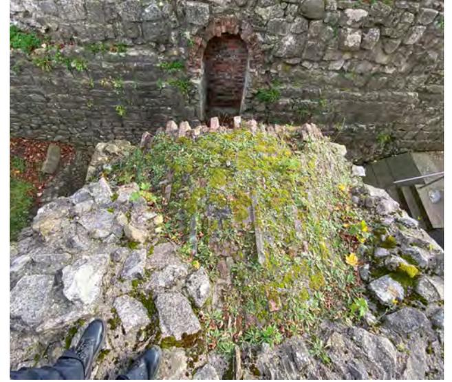
Vegetation and failing mortar and spalling brick to barrel vault
