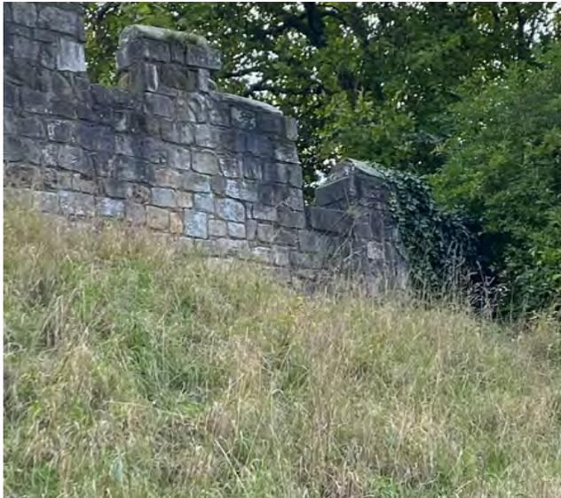
Missing section of merlon
