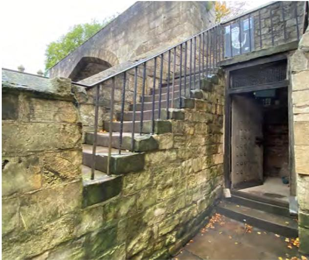
Fractured stones to steps from rust jacking to railings
