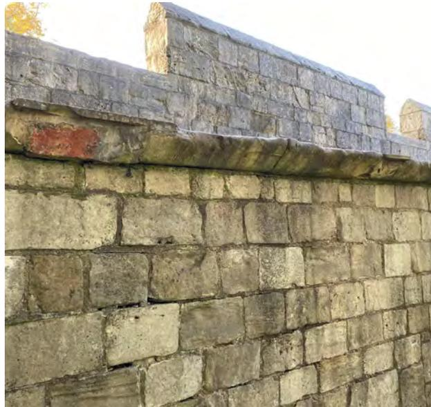
Poor repairs to edge stones of walkway
