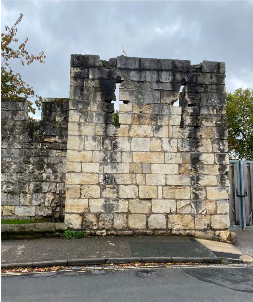
Exterior eroding stones from concentrated water movement from fractured stone to top course
