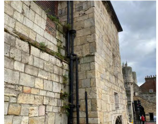
Rain water and soil pipes to north western elevation causing water ingress
