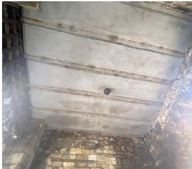
Rusting steel and concrete structure to carriageway
