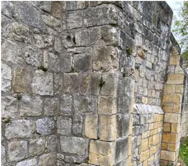
Structural movement to buttresses
