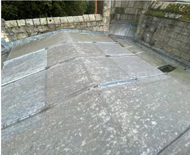
Leaking thin lead roof
