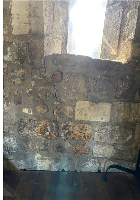
Internal cracking around windows with cloudy Perspex
