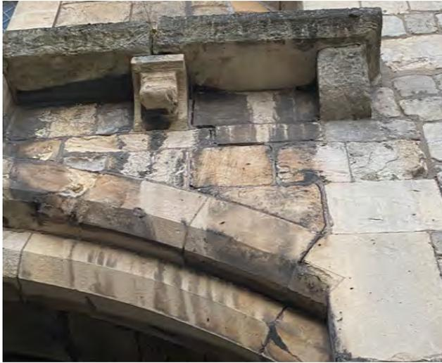
Crack to arch over carriageway on south side
