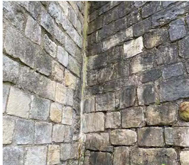
Structural movement at joint with west wall
