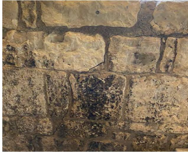
Cracks to east wall of top floor
