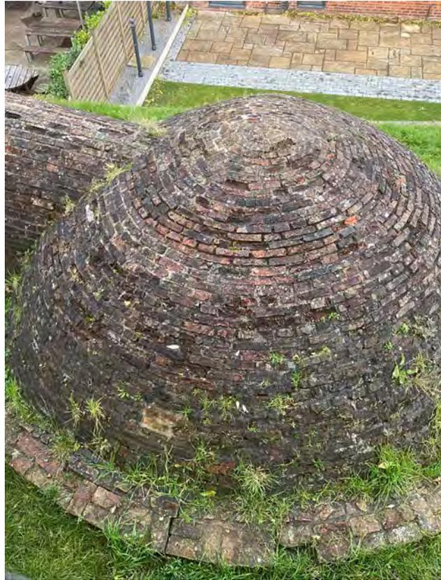
Failing mortar joints to uncovered exterior
