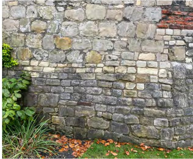
Open joints at low level externally
