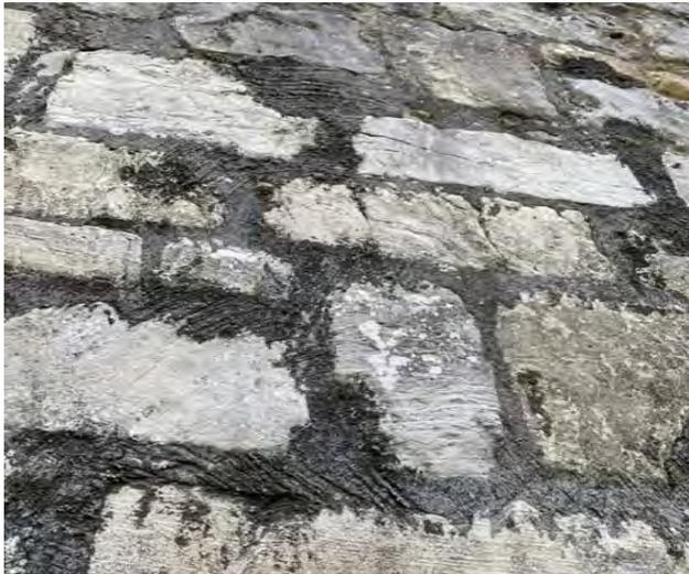
Dark cement mortar north of Multiangular tower
