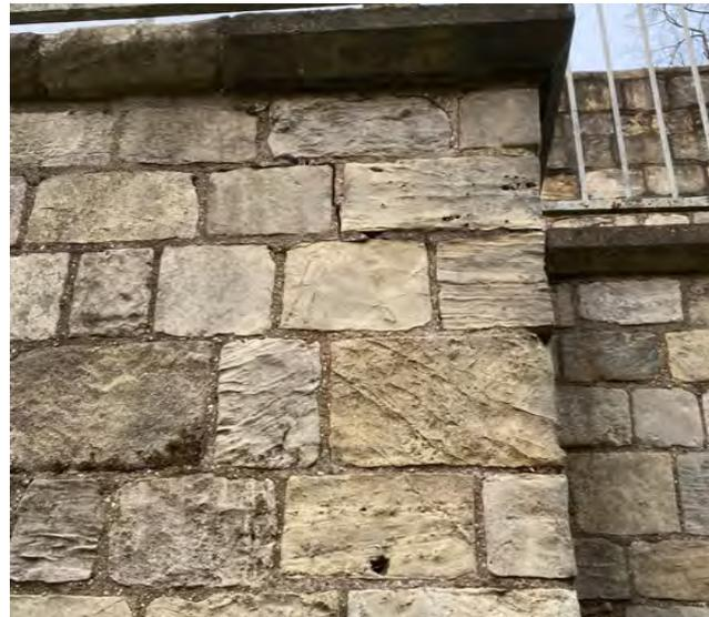
Movement crack to eastern walkway structure
