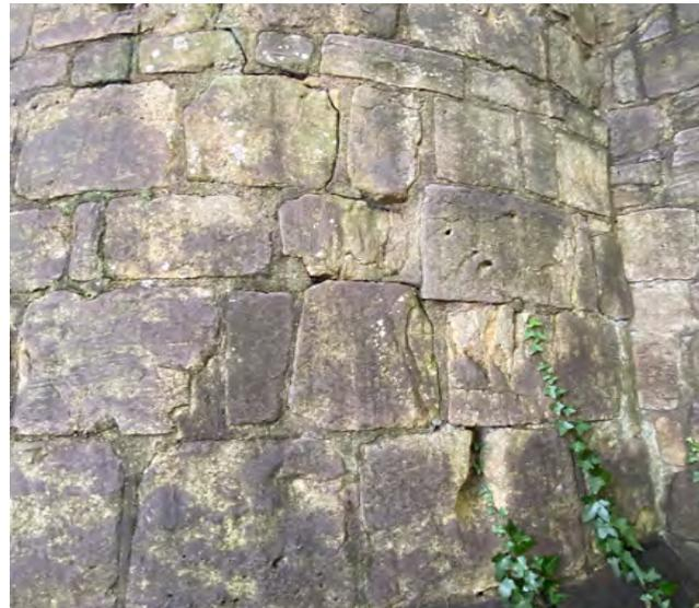
Vertical cracks to southern external elevation
