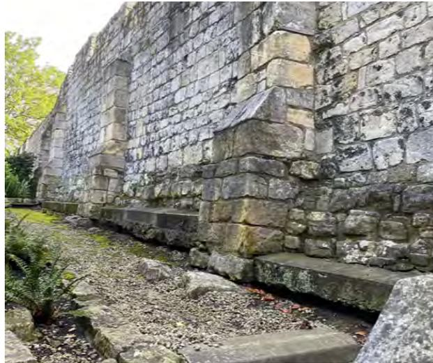
Erosion from under concrete footings
