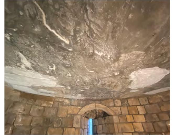
Internal ceiling showing water ingress
