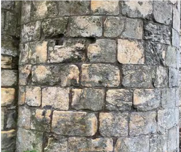
Cracking along mortar joints to exterior
