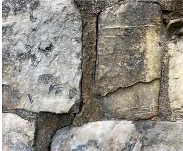
External structural movement cracks
