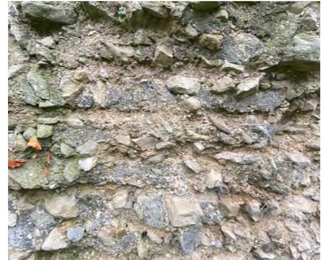
Exposed rubble wall actively falling away and eroding south of multiangular tower
