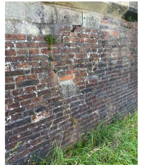
Vertical cracks through infill structure
