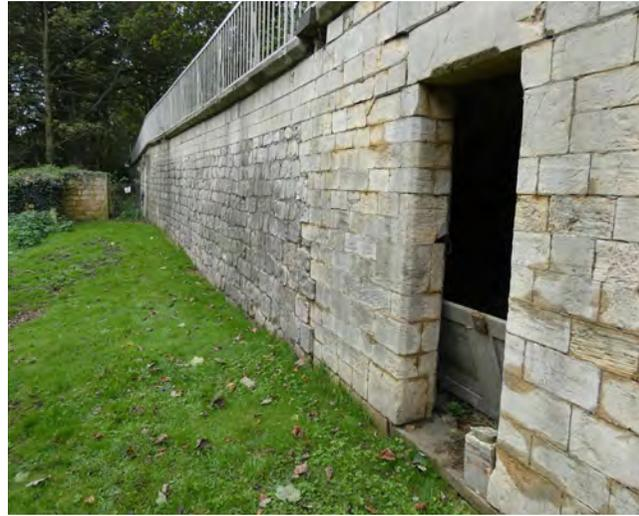
Entrance door, structural movement, fractured stones and failing mortar
