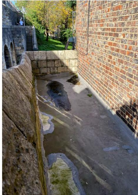
Failed asphalt roof next to eastern stair
