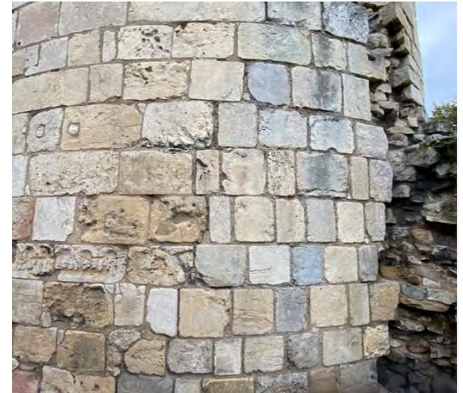
Structural movement cracks to south west corner
