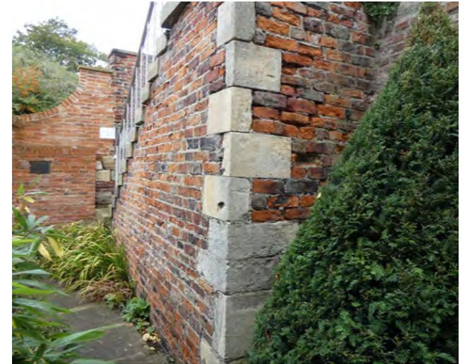
Open joints and raised stone landing slab away from supporting brickwork beneath
