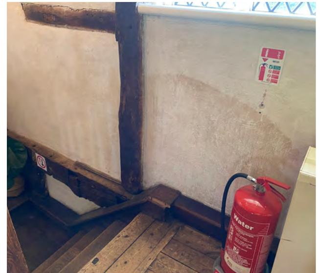
Water ingress to west elevation
