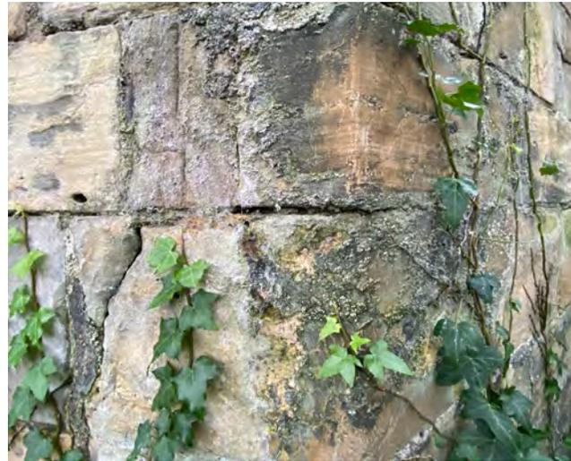
Salt movement and failing mortar from saturation
