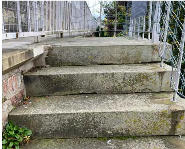
Fractured rotating top stone landing slab with cramp and cracks
