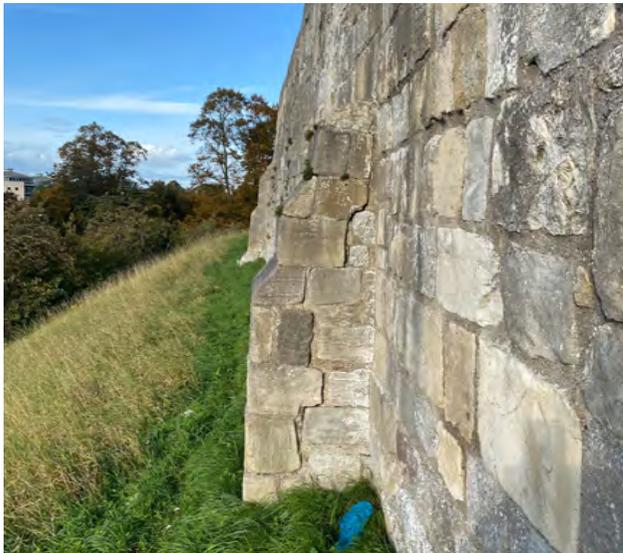
Structural movement to buttress between Tower 15 and 16
