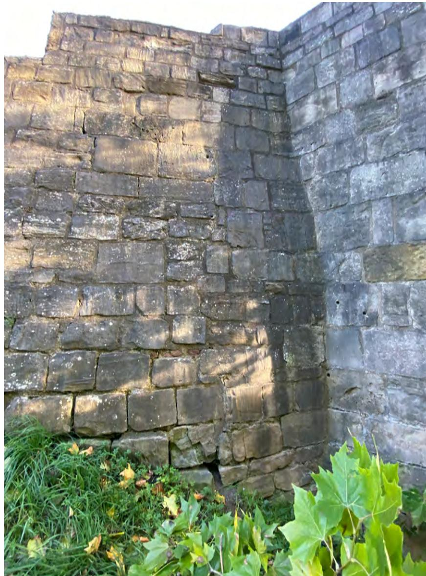
North west elevation open joints at low level
