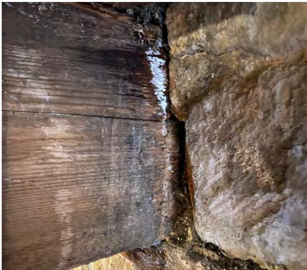
North west primary timber beam rotten within masonry pocket
