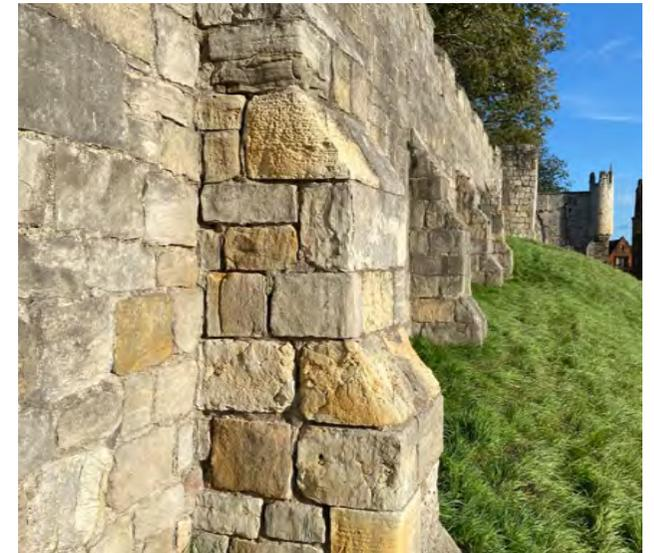
Structural movement to buttresses between Micklegate Bar and Tofts Tower
