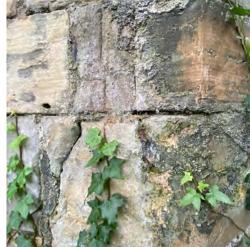
Salt movement and failing mortar from saturation
