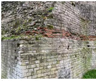
South internal corner with open core masonry
