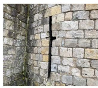
Structural movement to joint with east wall
