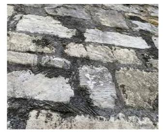
Dark cement mortar north of Multiangular tower
