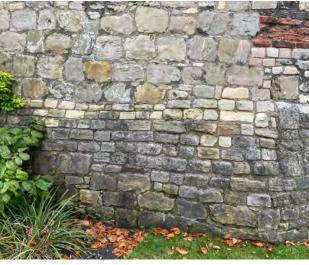
Open joints at low level externally
