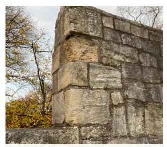
Eroding stone to merlon
