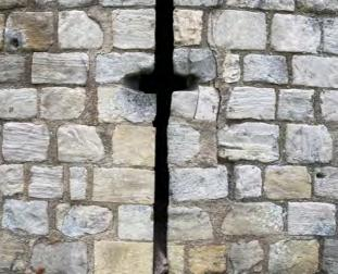
Fractured stones to perimeter of arrow slit
