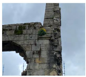
Structural movement to gable junction with wall
