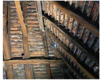
Holes in clay tile roof and rotting timber roof structure
