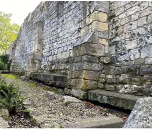
Erosion from under concrete footings
