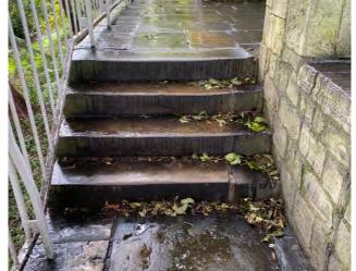
Movement cracks and seperation at steps
