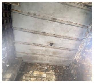
Rusting steel and concrete structure to carriageway
