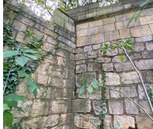
Movement cracks to wall junction north of tower
