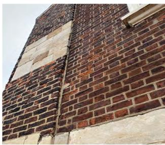
Open joint to west elevation
