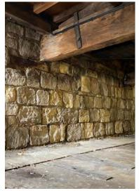
**3.11** Water ingress and saturation **3.12** Open joints
