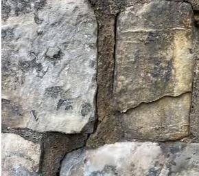
External structural movement cracks
