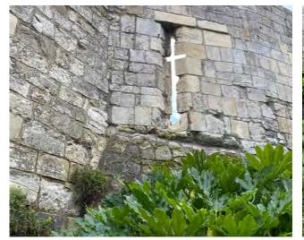
Failing cementitious mortar to north junction
