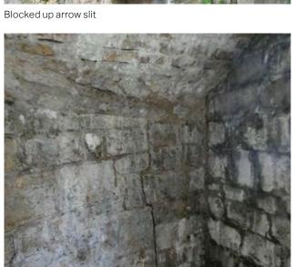
Structural movement to internal walls
