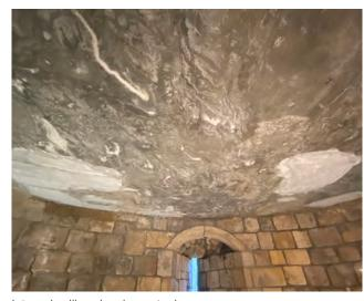
Internal ceiling showing water ingress
