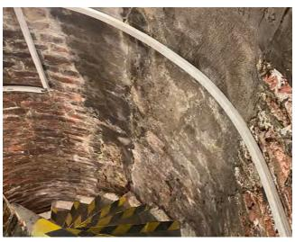
Internal water ingress through cementitious render to spiral stairs from external down pipes
