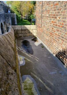
Failed asphalt roof next to eastern stair
