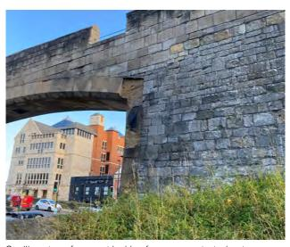
Spalling stone from rust jacking from concentrated water
