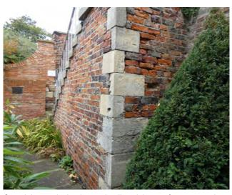
Open joints and raised stone landing slab away from supporting brickwork beneath
