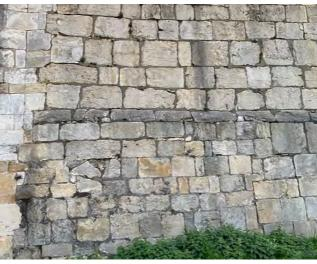
External wall by Fishergate Postern Tower with failing mortar joints
