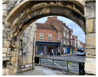
Erosion of stone from water getting trapped behind sulphuric crust
