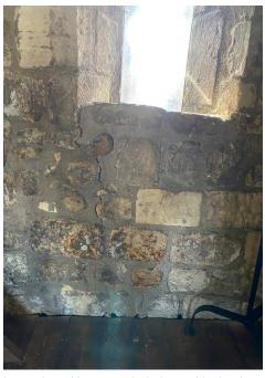
Internal cracking around windows with cloudy Perspex
