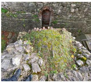
Vegetation and failing mortar and spalling brick to barrel vault
