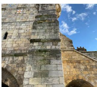
Structural movement cracks running up tower
