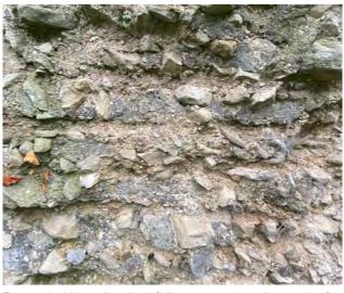
Exposed rubble wall actively falling away and eroding south of multiangular tower
