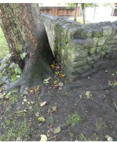
South elevation Tree causing structural movement to wall and IT A Movement crack
