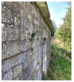
Mortar joint below edges stones moving outwards
