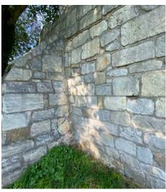
Structural movement to buttress on 560 chainage
