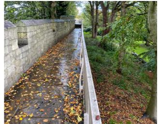
Bending railings with no movement joints
