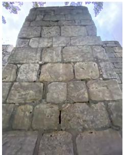
Structural cracks and open joints to southern elevation
