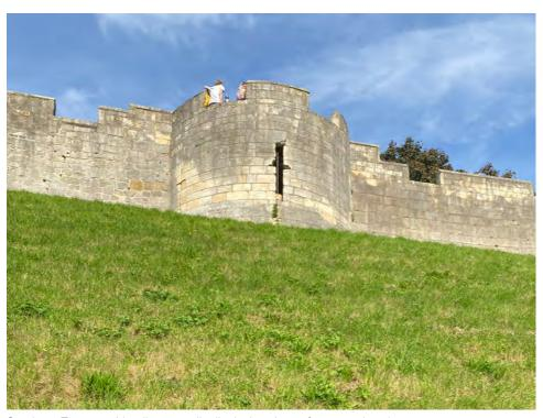
Section 3 Tower 7, with adjacent walls displaying signs of cannon shot damage
