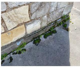
Missing lead and failing junction between asphalt and walls
