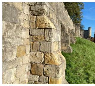
Structural movement to buttresses between Micklegate Bar and Tofts Tower
