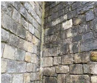
Structural movement at joint with west wall
