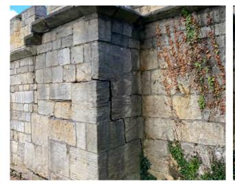
Cracking below steps and railings
