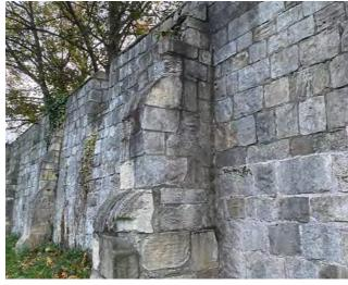
Missing masonry from buttress east of Robin Hood Tower
