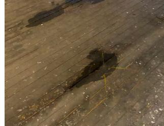
Multiple areas of water ingress from roof onto timber structure below
