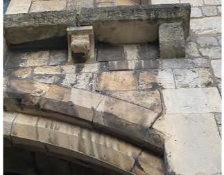
Crack to arch over carriageway on south side
