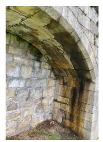
**3.15** Salt Movement and Saturated Masonry
