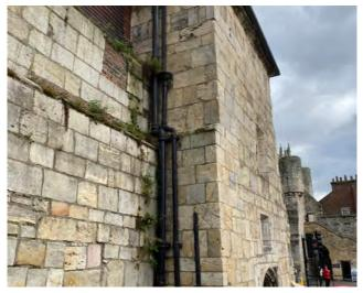
Rain water and soil pipes to north western elevation causing water ingress
