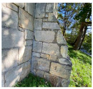
Structural movement to buttress 25m chainage
