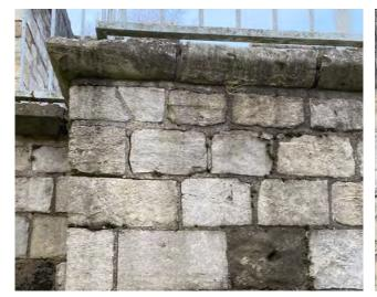
Cracking and open joints to western walkway structure
