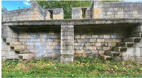
Steps built over with structural movement to central pier
