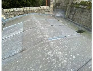
Leaking thin lead roof
