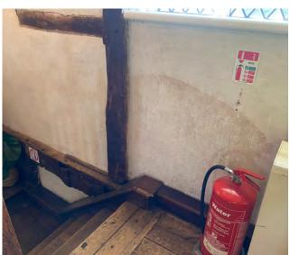
Water ingress to west elevation
