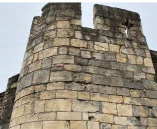
High level cracking and movement below crenel sill
