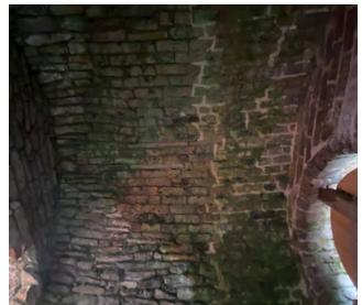
Structural movement cracks to brick barrel vault
