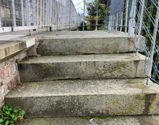
Fractured rotating top stone landing slab with cramp and cracks
