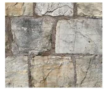
Movement crack to south elevation
