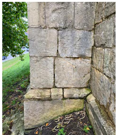
Movement crack to north side
