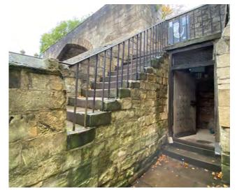
Fractured stones to steps from rust jacking to railings
