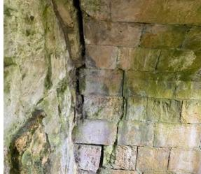
Joint failure between Victorian and Medieval structure
