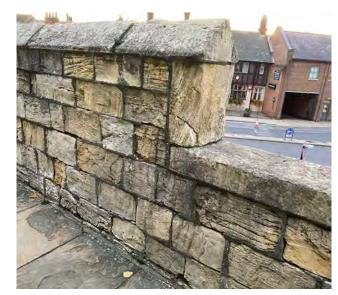
Fishergate Postern Tower end poor parapet wall condition
