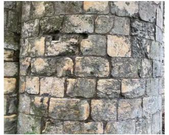
Cracking along mortar joints to exterior
