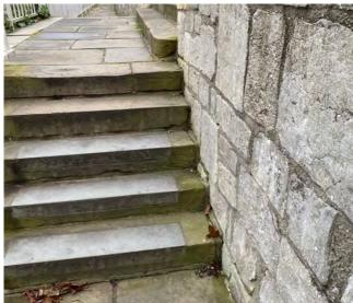
Walkway steps, enlarging joints against parapet wall
