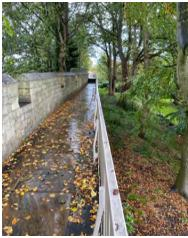
**3.06** No movement joints to railings **3.07** No tying in of masonry joints **3.08** Edge stones with no drip
