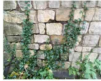
Saturated masonry at low level with failing mortar
