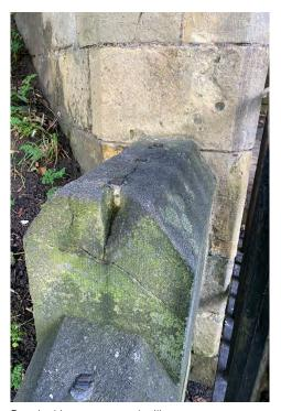
Rust jacking to removed railings
