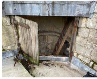
No covering to access hatch to roof which is allowing water in
