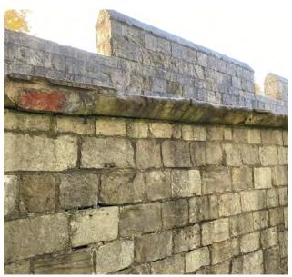
Poor repairs to edge stones of walkway
