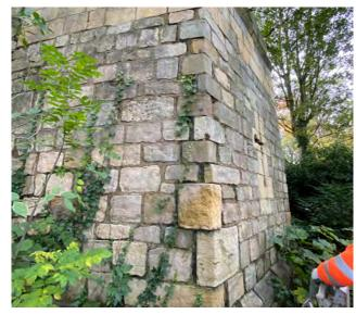
Separation of masonry around the quoins of tower
