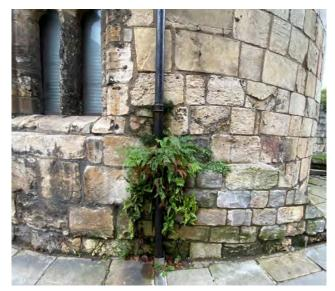
Leaking rain water pipe
