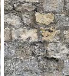
Diagonal cracking to wall on the west side of tower
