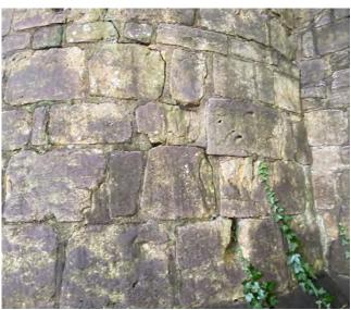
Vertical cracks to southern external elevation
