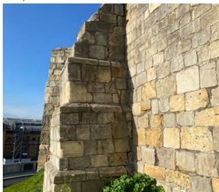
Structural movement to buttress next to Tofts Tower
