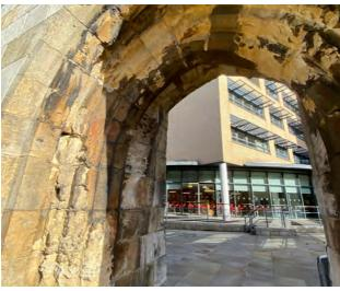
Heavily weathered stones to Victorian pedestrian arch between railway arches
