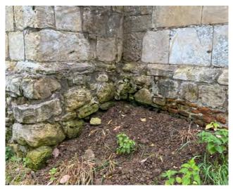
Rubble foundations are failing
