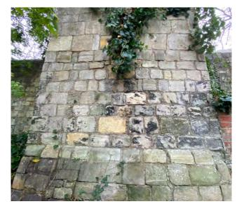
Vegetation growth and open joints to west elevation
