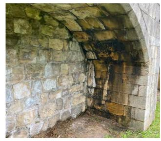
Saturation to interior of internal arches
