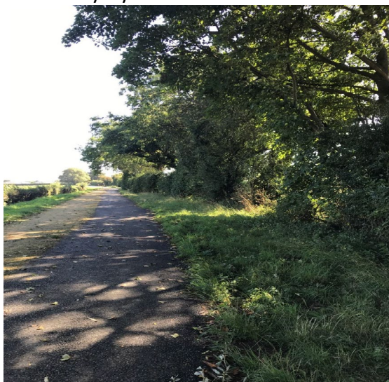
Figure 2 Moor Lane on northern edge of project area
