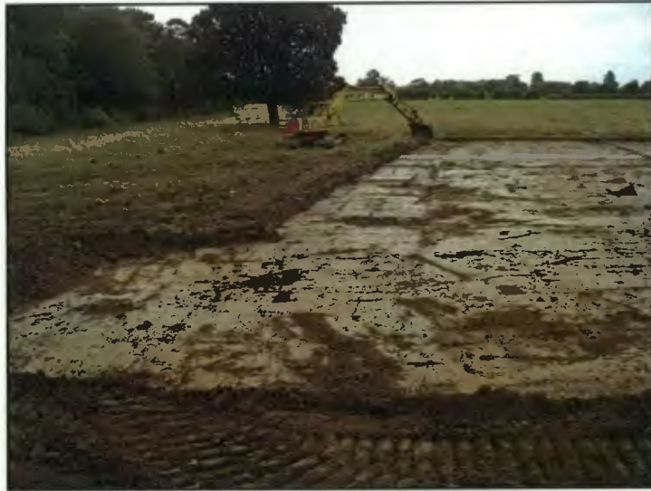
Plate 1. General site shot during topsoil strip, looking north
