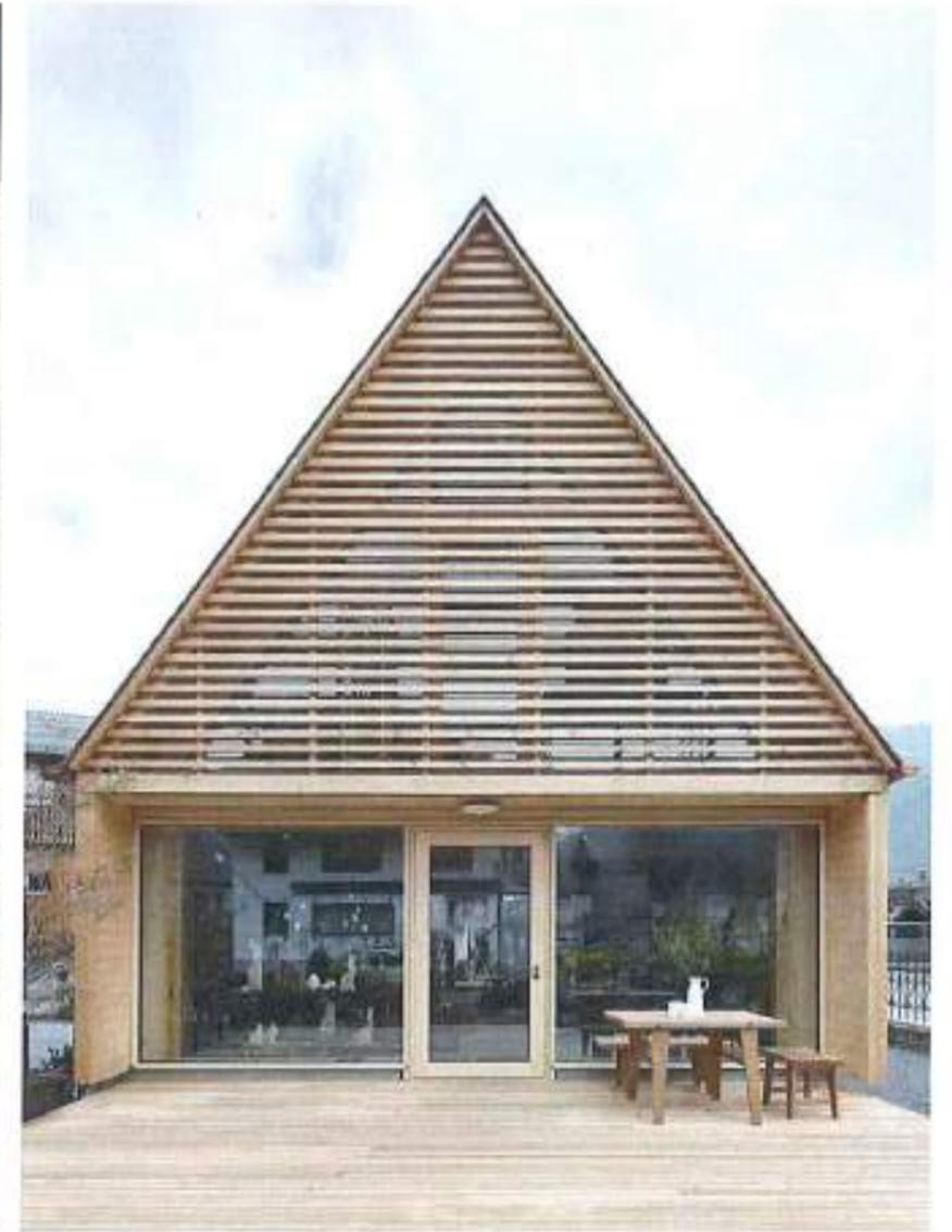
EXTERIOR REFERENCES: TRANSLUCENCY IN UPPER STOREY CLADDING. LOWER SECTION GLAZED
