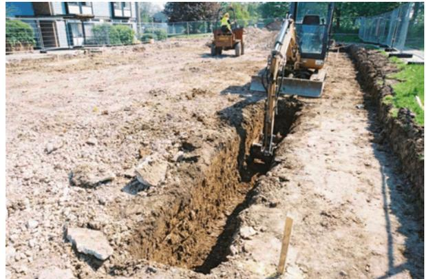
**Plate 1** Foundations under excavation
