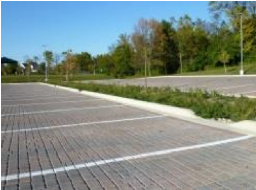
Figure 4: Example of SuDS integrated into a development (Permeable paving York St Johns University))
