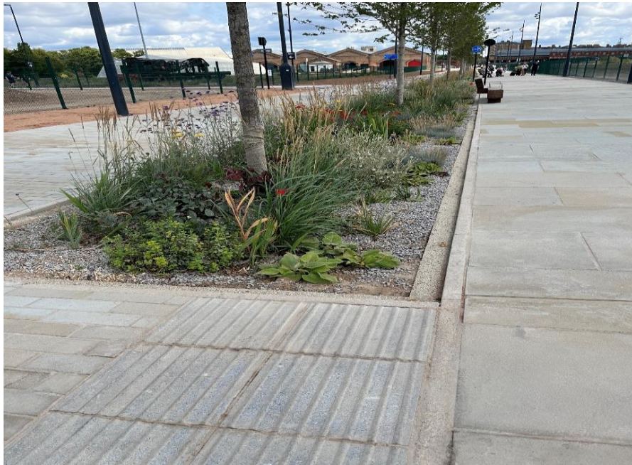
Figure 3: Example of SuDS integrated into a development (Raingardens - York Central Main Spine Road)
