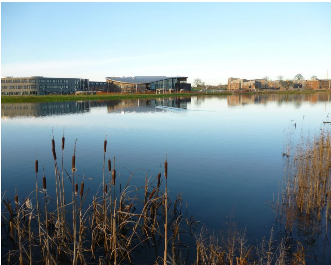
Figure 2: Example of SuDS integrated into a development - (Heslington East University Campus central lake attenuation basin with permanent body of water)
