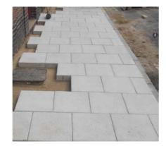
Grey Saxon paving in the process of being laid on Priory Street as a stretcher bond
