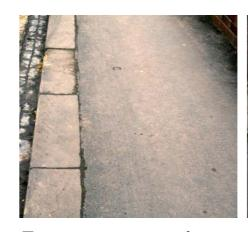
Tarmac pavement surface used to good effect with broad-top English Pennine sandstone kerbing
