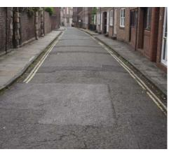
Asphalt carriageway surface in Aldwark with mixed aggregate inclusions
