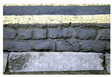
Brick drainage channel parallel to the kerb and carriageway
