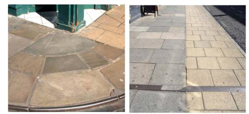
Well though out approach to laying riven flags at a corner - note the original cast iron kerb, used to protect the pavement edge
