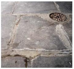
Wide joints in riven English Pennine sandstone poorly pointed with cement mortar
