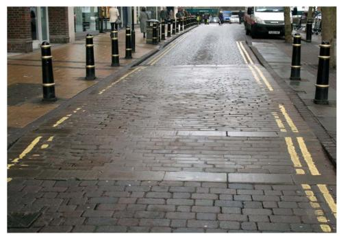
Raised table on Parliament Street consisting of English Pennine sandstone setts with pre-cast brick paviours on either side
