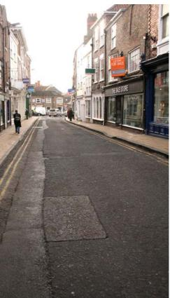
Colliergate with narrow footways surfaced in small square pre-cast Saxon flagstones and a poor quality carriageway surface
