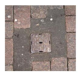
Repair work by utility contractors using cement rather than original brick paviours
