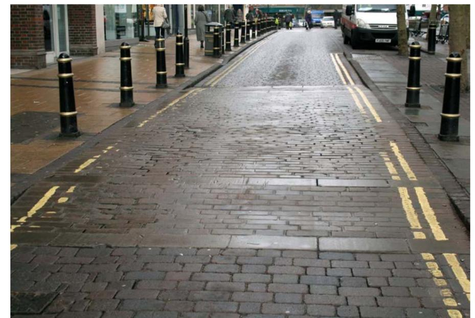
*Raised table on Parliament Street consisting of English Pennine sandstone setts with pre-cast brick paviours on either side*
