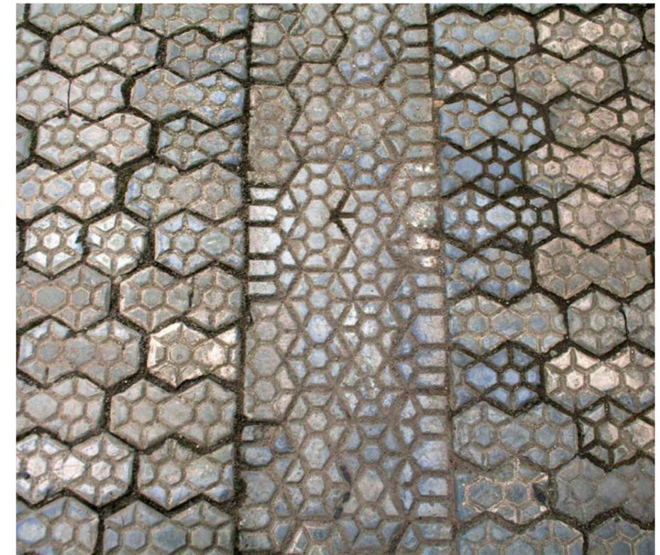
**Stable paviours in Southbank with a carefully laid drainage channel running through.**
