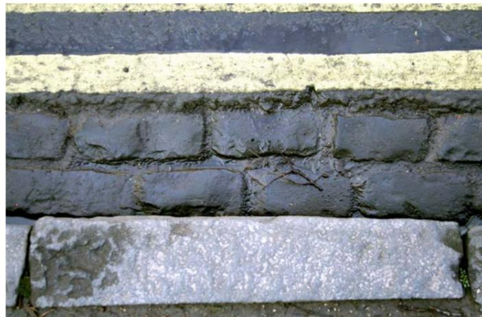
Brick drainage channel and granite kerb with neatly laid asphalt.
