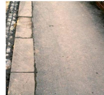
Tarmac pavement surface used to good effect with broad-top English Pennine sandstone kerbing
