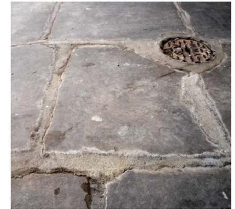
**Wide joints in riven English Pennine sandstone poorly pointed with cement mortar**
