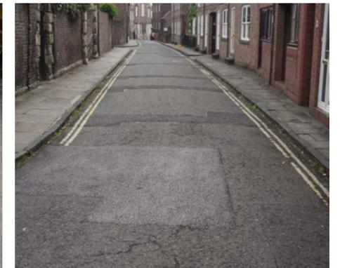
Asphalt carriageway surface in Aldwark with mixed aggregate inclusions
