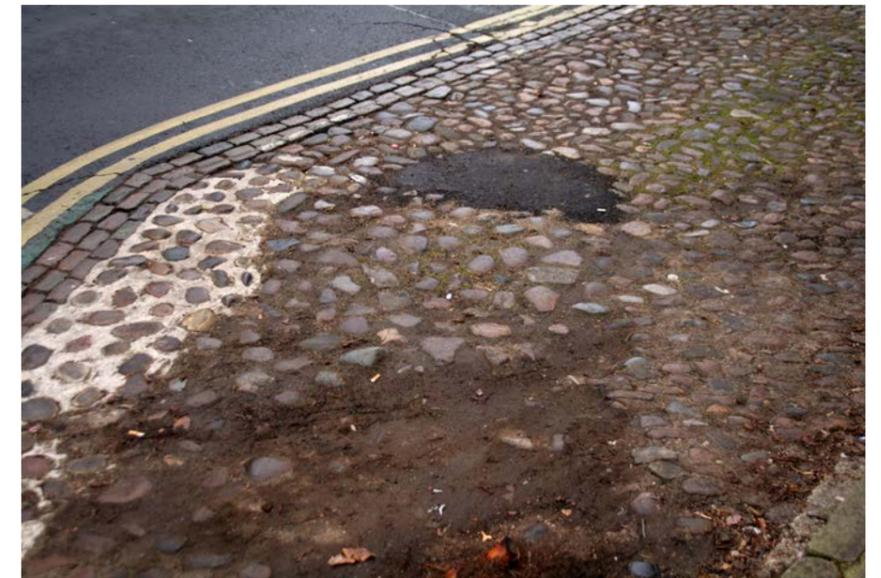
*Cobbles on Blossom Street with contrasting reinstatement (white cement) and repair (asphalt)*
