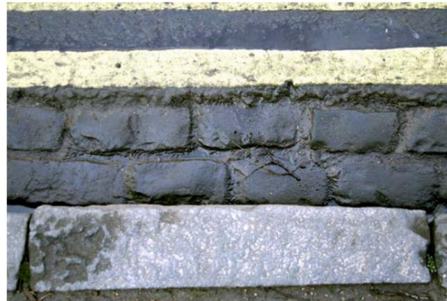
*Brick drainage channel parallel to the kerb and carriageway*
