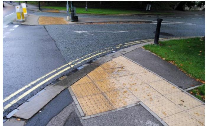
**Excessively wide junction splay and incorrect tactile paving installation (tail implies controlled crossing)**
