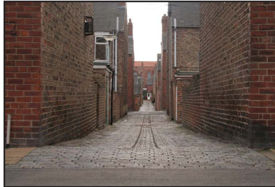
A particularly well preserved section of historic stable paviours on a side lane in Southbank
