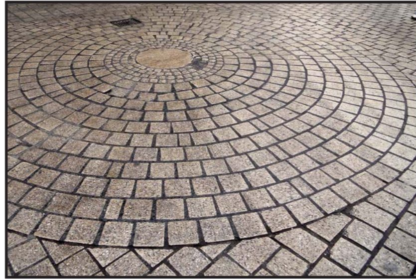
A fine example of the decorative use of blanc-de-bierge setts in Spurriergate
