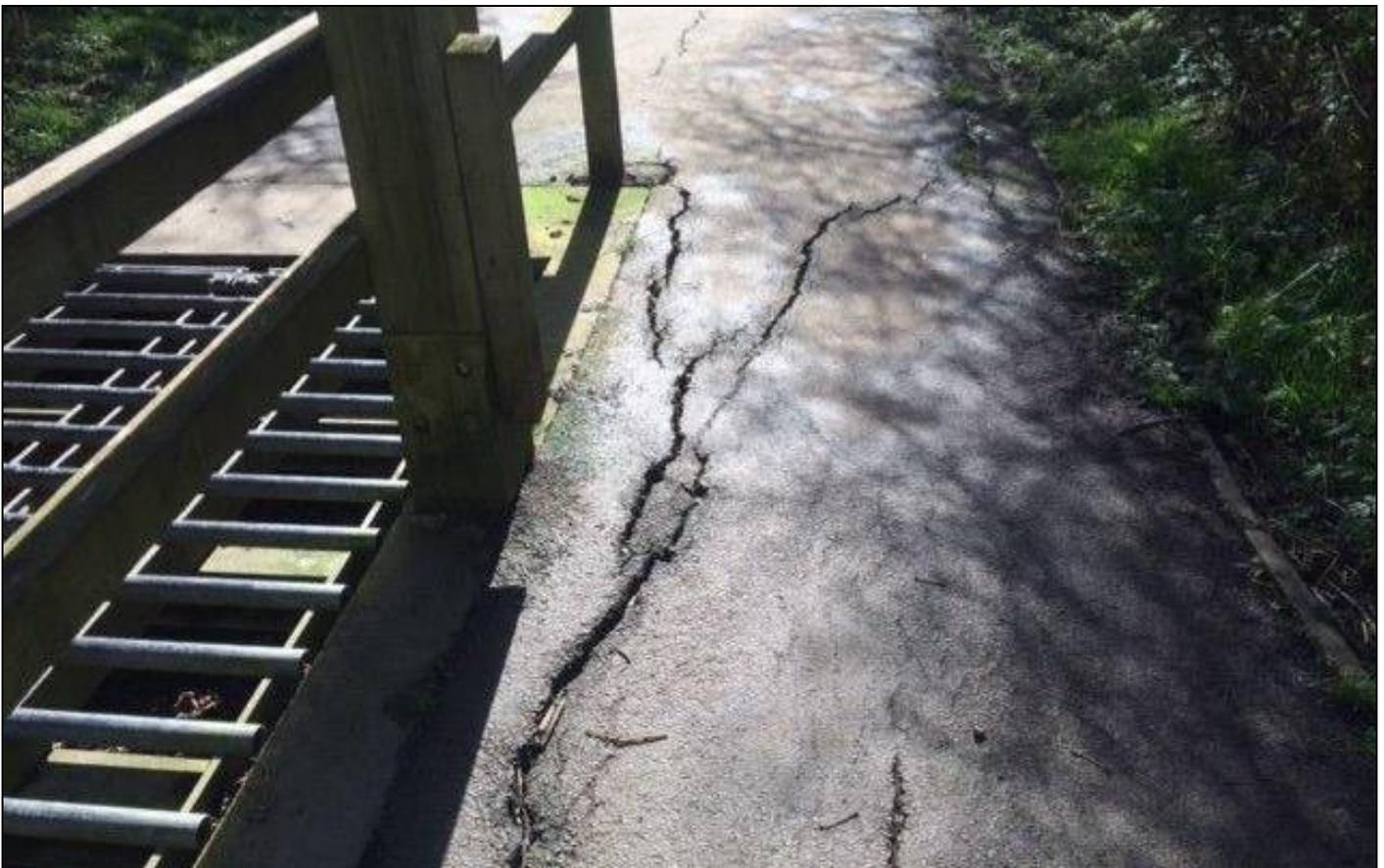
Cracking to path adjacent to access control
