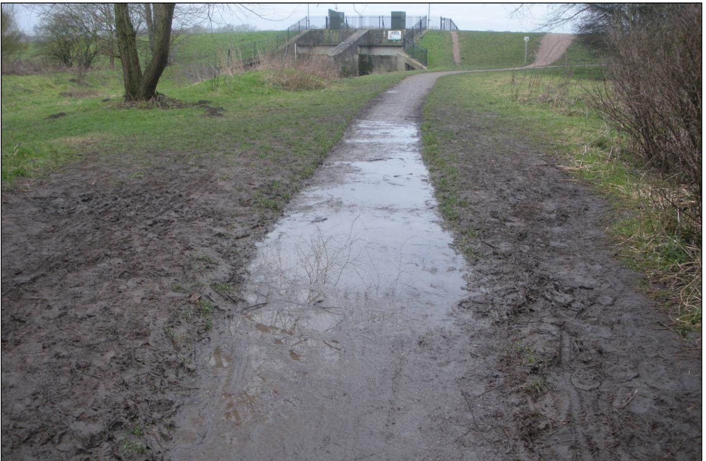
Flooding to path as a result of poor drainage
