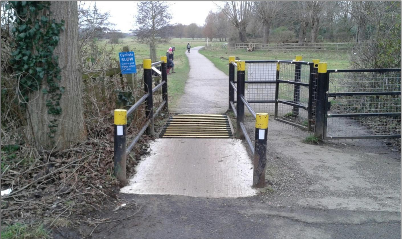
Example of recently improved access barrier elsewhere in York with anti-skid surface applied to cattle grid and surface improvements on approaches
