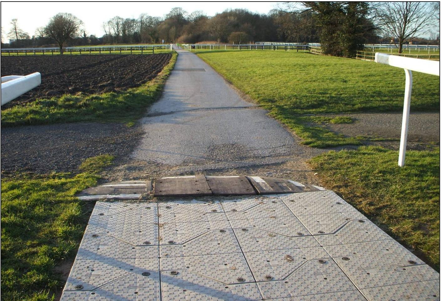
Poorly-aligned ramps onto temporary roadway where the route crosses York Racecourse
