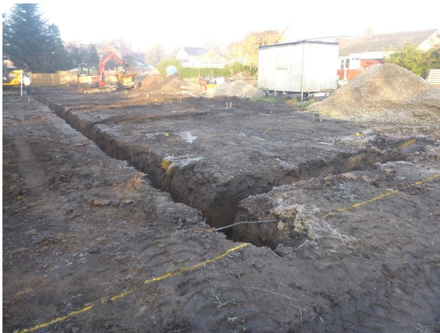
Plate 1 Overview of site
