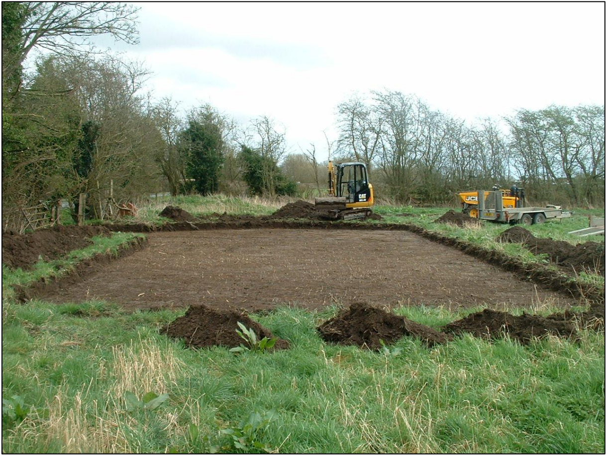
Figure 3. View of completed excavation looking east.
