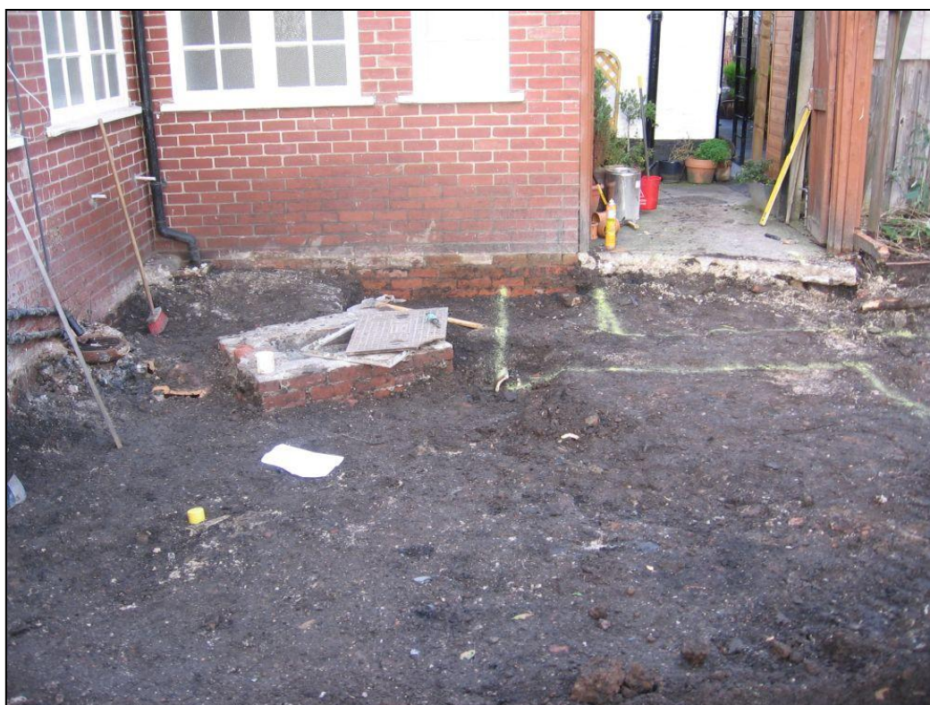
Plate 1 General view of site, looking north-east
