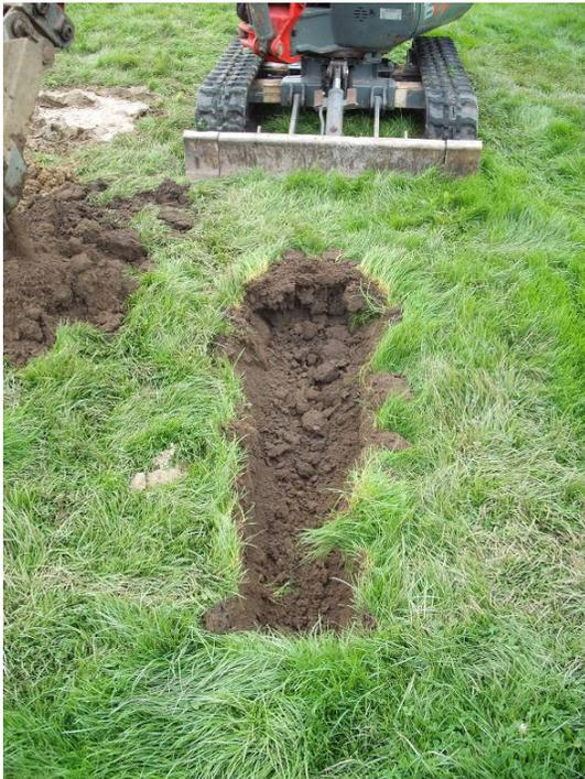
Plate 4: Opening ground on Trial Pit 2
