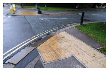
Excessively wide junction splay and incorrect tactile paving instalation (tail implies controlled crossing)
