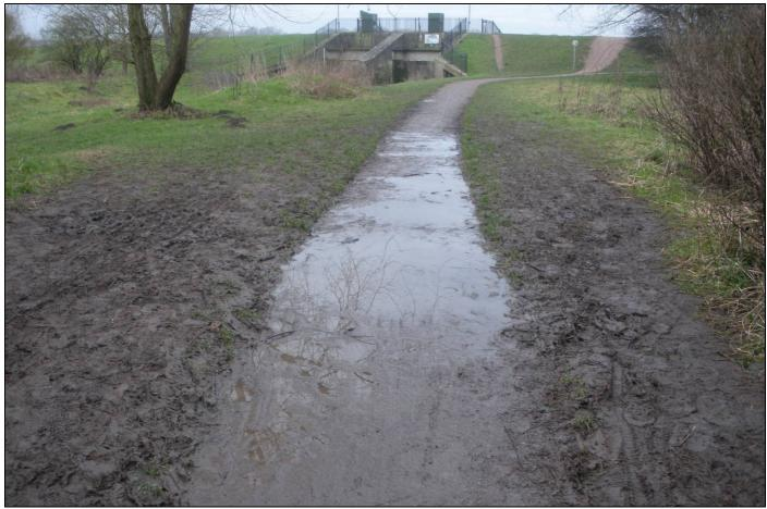
Flooding to path as a result of poor drainage
