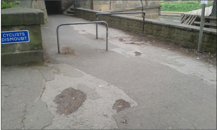
Damage to path surface on NCN 65 adjacent to Scarborough Bridge
