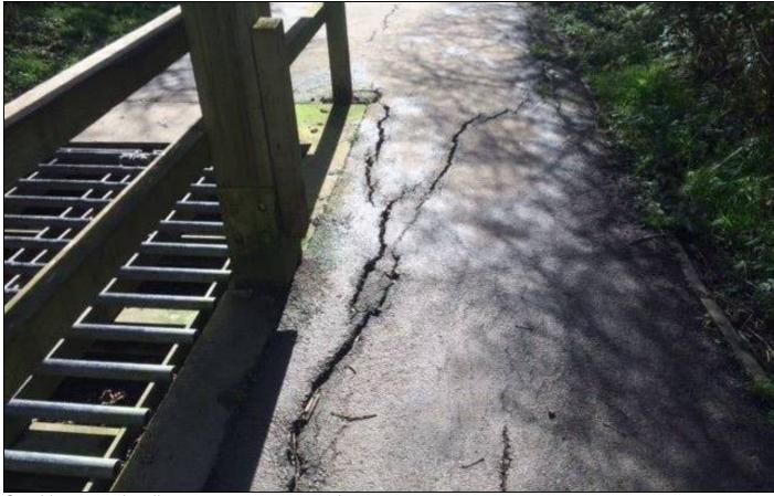
Cracking to path adjacent to access control
