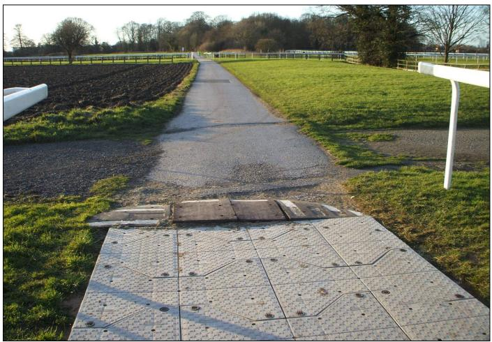
Poorly-aligned ramps onto temporary roadway where the route crosses York Racecourse
